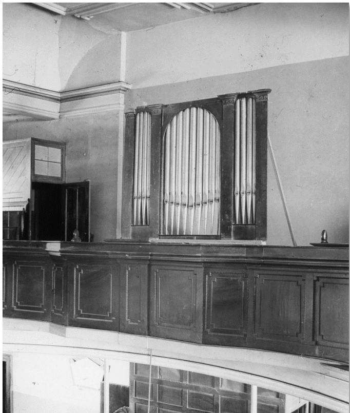
The 1828 pipes in their original location before the major rebuilding phase of the 1930s
