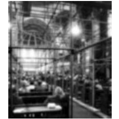
1981 - 1984 St. John's Church Restoration Project - Picture Gallery (ASJ2023.13)
