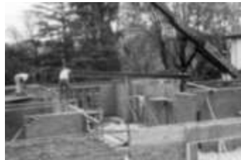
1970s Parish Centre construction - Picture Gallery (ASJ2023.12)
