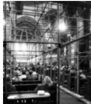
1981 - 1984 St. John's Church Restoration Project - Picture Gallery (ASJ2023.13)
