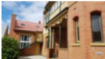
1893 to 1950 - St. John's Mission House - Picture Gallery (ASJ2023.3)
