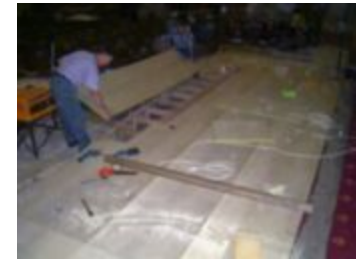
2003 - Building of dais - Picture Gallery (ASJ2023.14)
