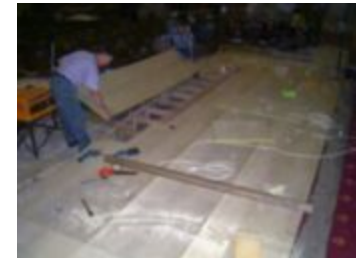
2003 - Building of dais - Picture Gallery (ASJ2023.14)
